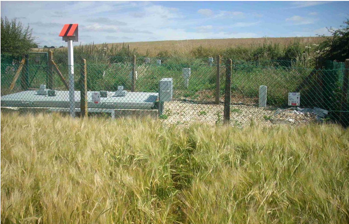
Photograph 3.1: An Existing Valve Enclosure and Flight Marker Post
